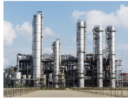
Oil and gas pipeline surveillance
